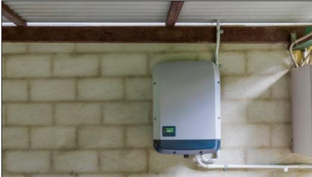
Figure 9. Behind-the-meter battery storage system
